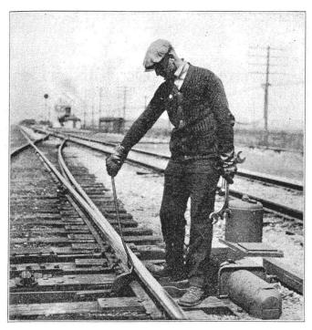
R. J. Walimire, maintainer, testing the adjustment of a switch
